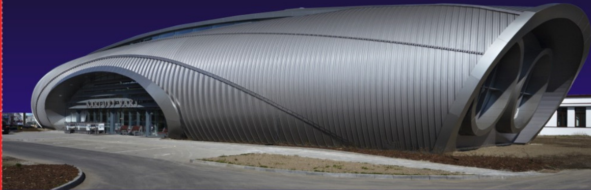
Karlovy Vary Airport Terminal, Czech Republic
